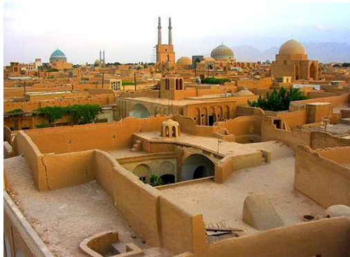
The roofscape of Yazd city
