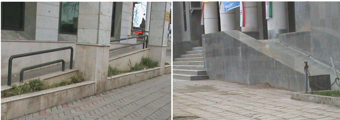
Pictures 6 and 7: A not standard ramp to a bank.
