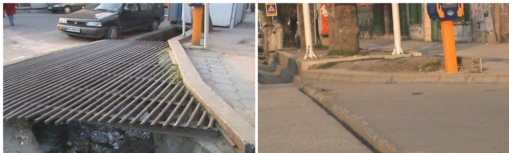
Figures 9 and 10: The junction point between pedestrian and street should be flat but in these pictures we are faced to some levels.
