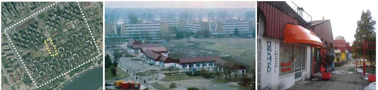
Figure 3: First shopping centers built in New Belgrade - a/ the position in the block; b/ and c/ the built structure.
