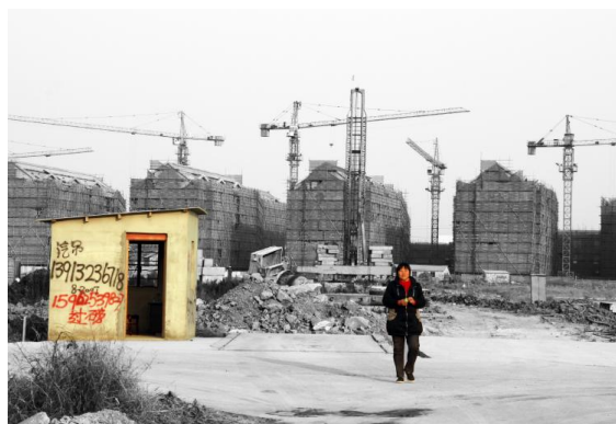
Fig. 4: Construction Site near Shanghai
