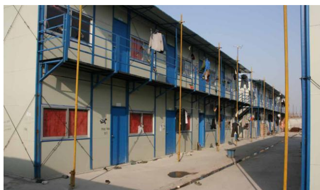
Fig. 7: Taicang construction site visit
