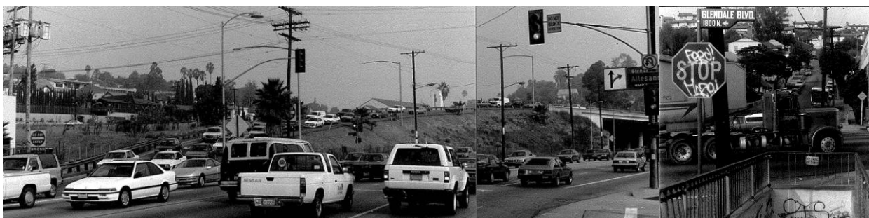
Fig. 5: The End of the Glendale Freeway in 1990 – a steep off-ramp merges onto Glendale Boulevard towards Downtown L.A. Dangerous and unattractive underpaths are the only safe crossing passages for pedestrians.
