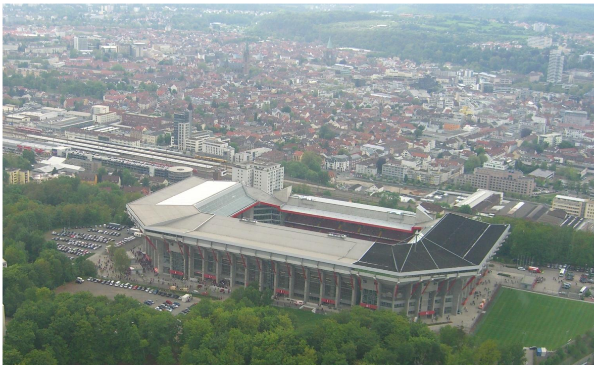
Fig. 1: View on the Fritz Walter Soccer Stadium in Kaiserslautern from the South (source: REPKA project).
