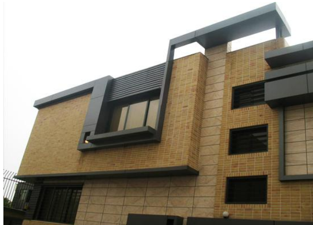
Fig. 18: Mostaghimi House, Ali Ghahremanpour, 2006
