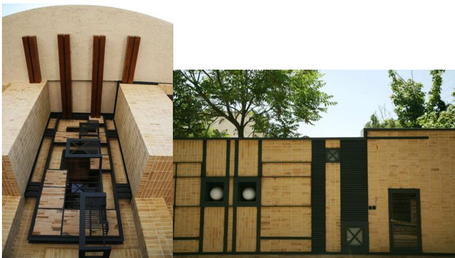
Fig. 13&14: Mostaghimi House, Ali Ghahremanpour, 2006
