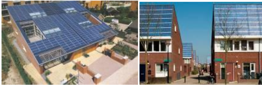
Figure 9 and 10: Experimental low energy houses in Nieuwland in Amersfoort, built in the early 1990s, demonstrated all kinds of techniques and systems. The sustainable residential area Nieuwland in Amersfoort consists of 4,500 houses. One thousand of them are covered with solar cells.
