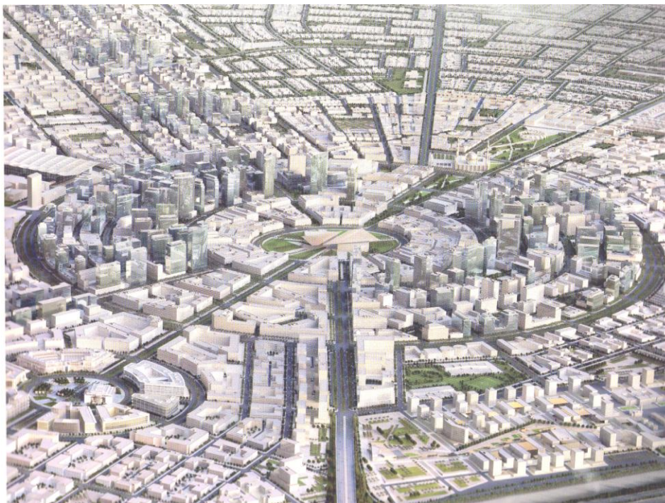
Figure 4: The 3D model of the main square in the capital district. Source: Source: The Abu Dhabi Urban Planning Council, 2007
