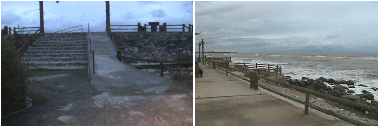
Picture 1: The ramp isn't standard and wheelchair users could not go to beach. Picture 2: There is no ramp in the beach.
