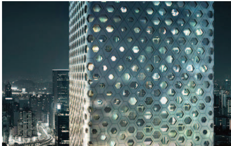
Fig. 9: the windows spreads in a random way to allow sun and wind to enter the building
