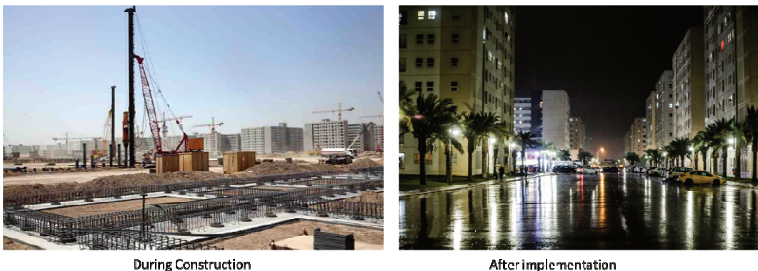
Fig. 4: Bismayah project during and after construction (National Housing Program, 2018)
