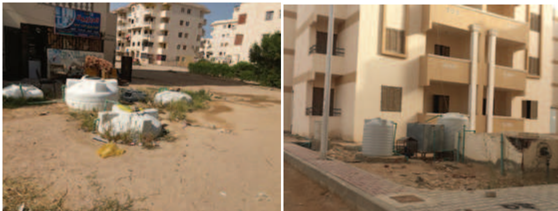
Fig. 9: water supply tanks - photos by author, 2018
