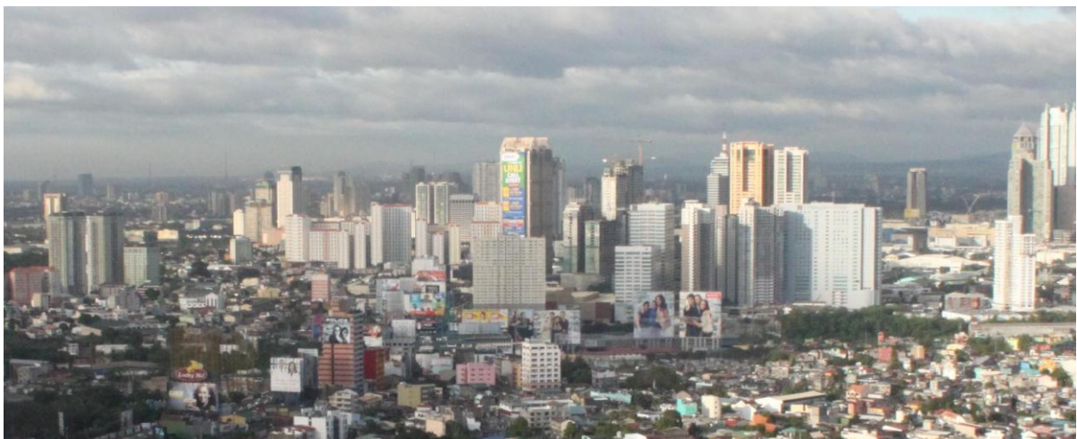
Image 8: Pioneer / Boni Avenue at EDSA. Emerging mixed-use cluster based on transit station of MRT line. Source: Stefan Rau.
