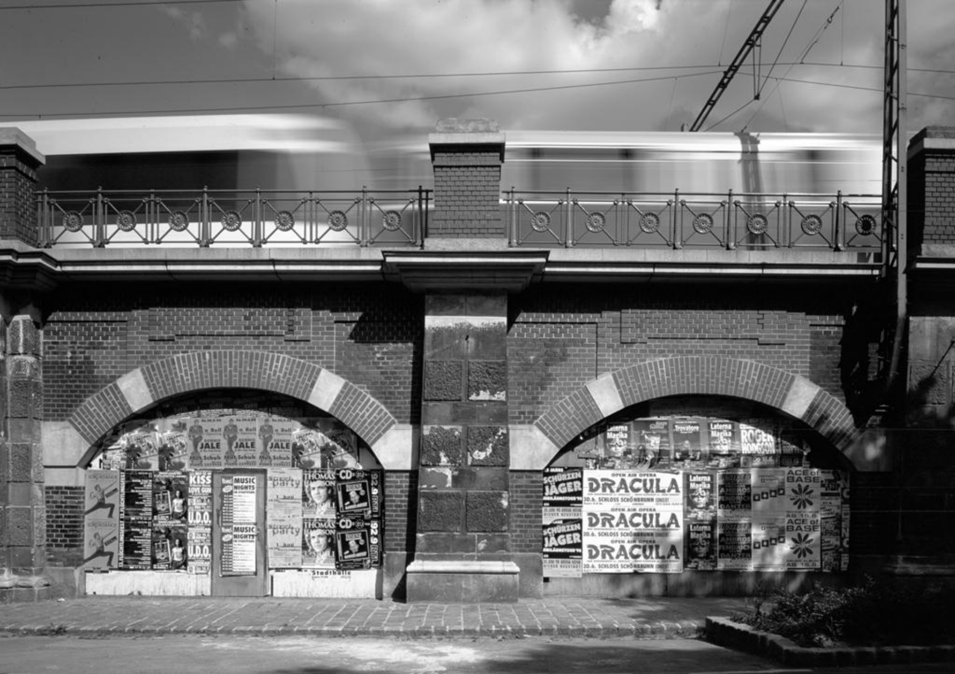
Closed arches form a barrier
