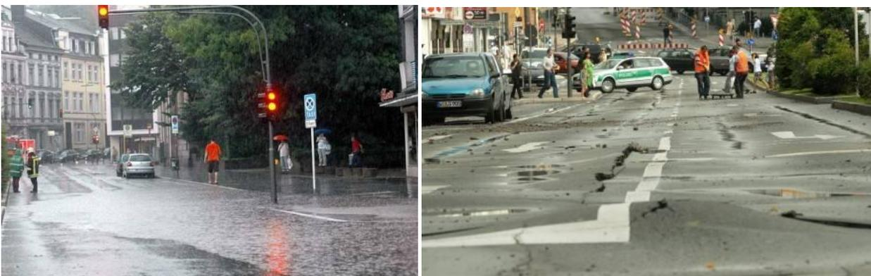
Figure 4: Damage due to uncontrolled storm water run-off.
