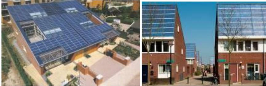
Figure 9 and 10: Experimental low energy houses in Nieuwland in Amersfoort, built in the early 1990s, demonstrated all kinds of techniques and systems. The sustainable residential area Nieuwland in Amersfoort consists of 4,500 houses. One thousand of them are covered with solar cells.
