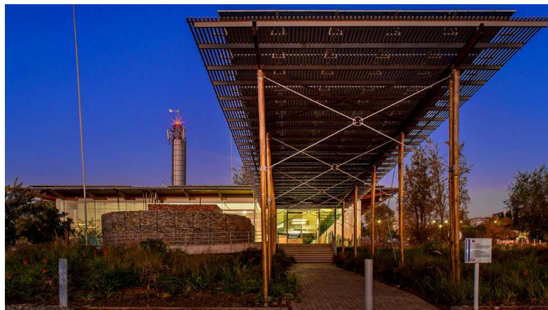
Fig. 5: Side view of Photovoltaic solar panels (Source: GLH Architects, 2011)
