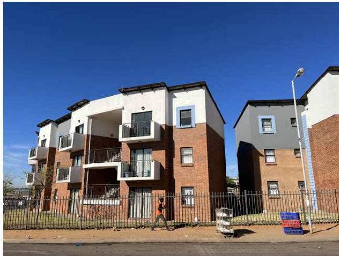
Figure 3: Middle-income rental flats in the low-cost households of Olievenhoutbosch Extension (Source: Author,2023).
